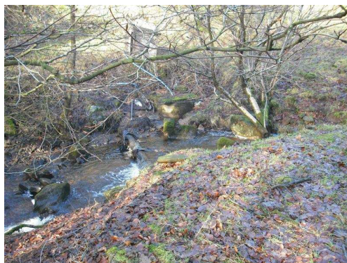
Figure 2 Weir constructed in channel
