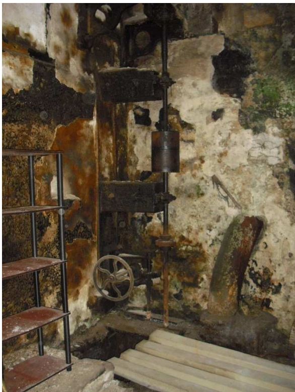
Figure 5 The turbine pit with some machinery above in situ
