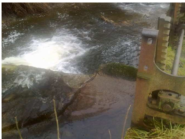
Figure 3 The sluice gate at the intake weir
