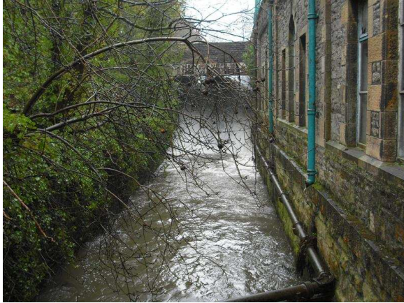
Figure 2 Intake weir from downstream
