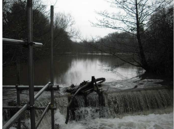
Figure 3 Existing intake channel above weir
