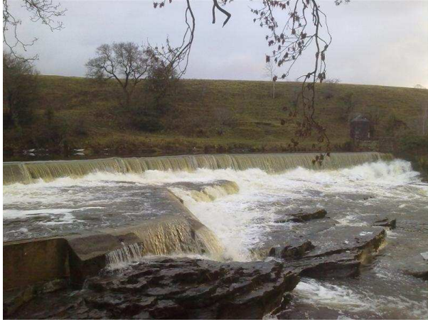
Figure 2 Weir from below showing sluice gates on the far side
