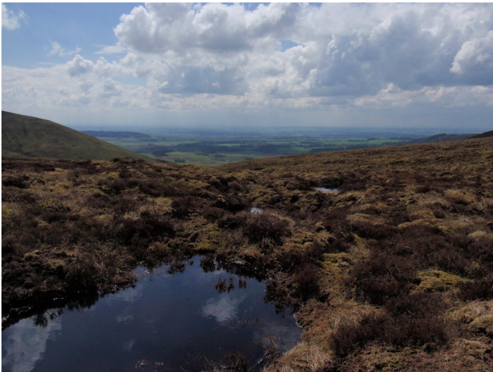
Gully at Fiendsdale Head re-profiled with check dams in place, May 2013
