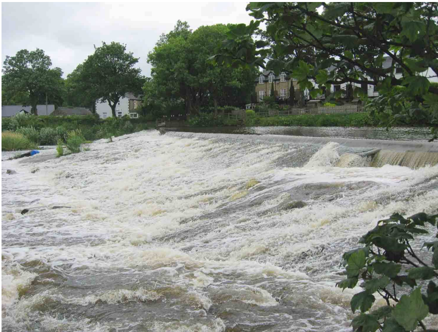
Figure 2 View of the weir from the south bank
