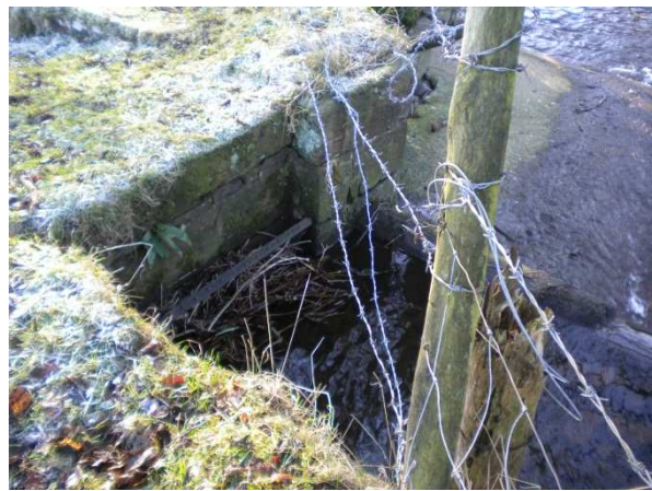
Figure 4 The intake with iron grate
