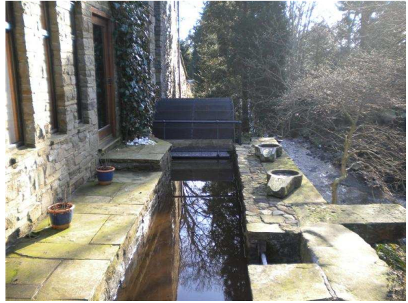
Figure 3 The headrace with the top of the mill wheel
