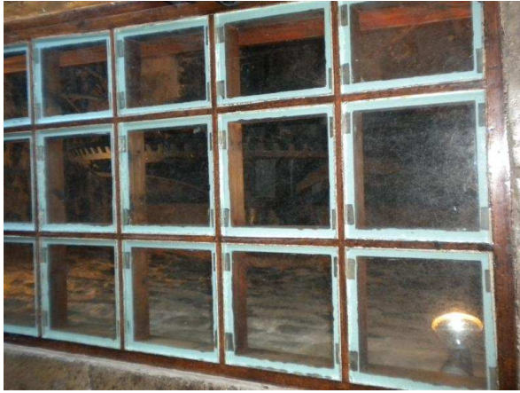
Figure 2 The remaining internal works
