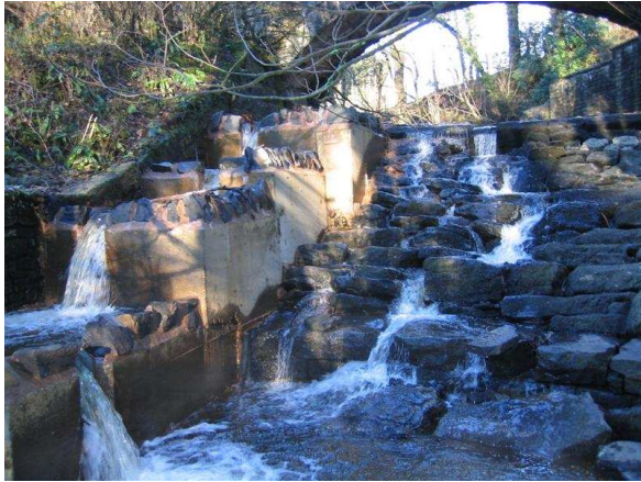
Figure 2 The weir and fishpass at Talbot Bridge
