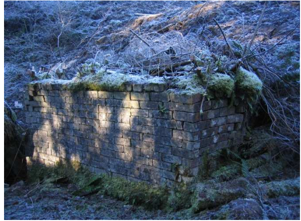
Figure 3 An old pump house
