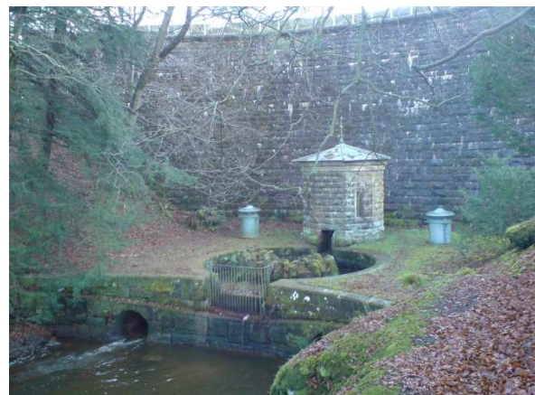
Figure 3 Lower outlet from dam
