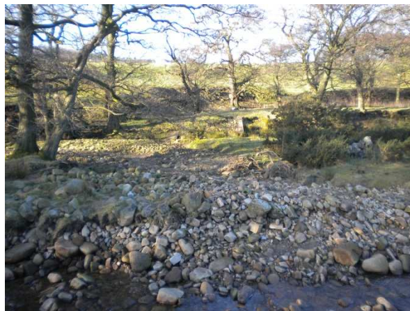
Figure 3 The position of the weir – now washed away
