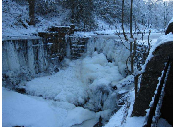
Figure 3 The weir face showing the overspill on the far left
