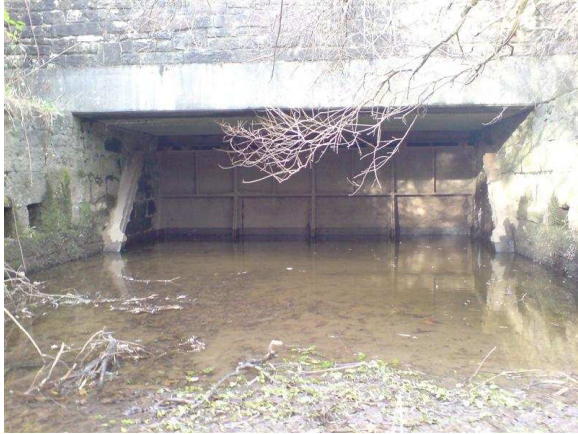
Figure 2 The sluice gate
