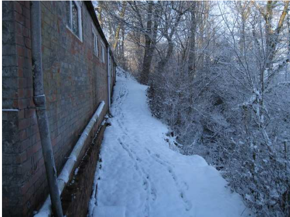
Figure 4 Looking along the leat or pipe route
