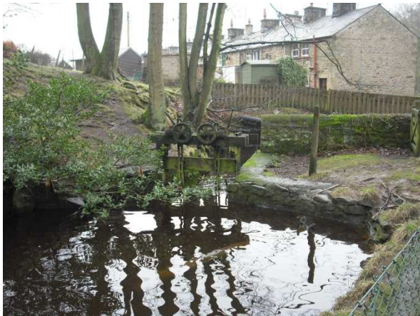
Figure 4 The mill upstream of the culvert
