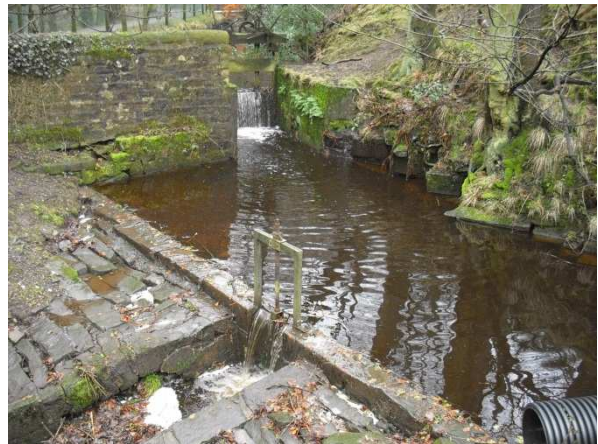
Figure 5 The basin at the culvert outlet
