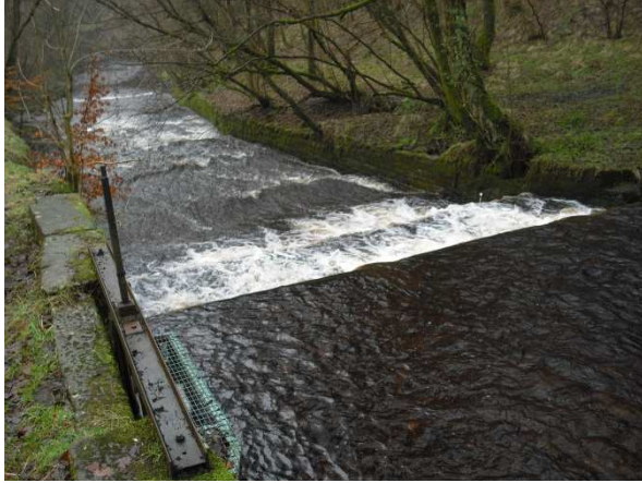
Figure 2 The weir and intake sluice
