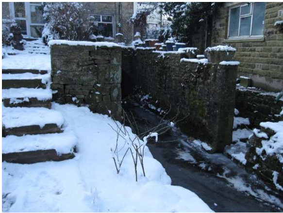
Figure 4 The potential powerhouse location above the youth hostel
