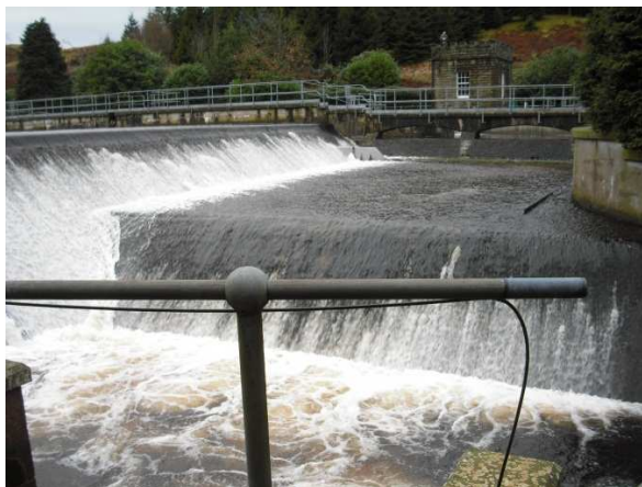
Figure 2 The series of weirs at the intake site
