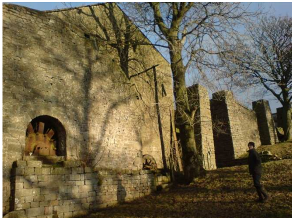
Figure 4 The stone columns supporting the wooden lade, or launder
