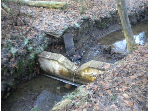
Figure 3 The v-notch measuring weir
