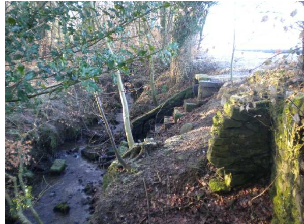
Figure 4 The outfall from the reservoirs
