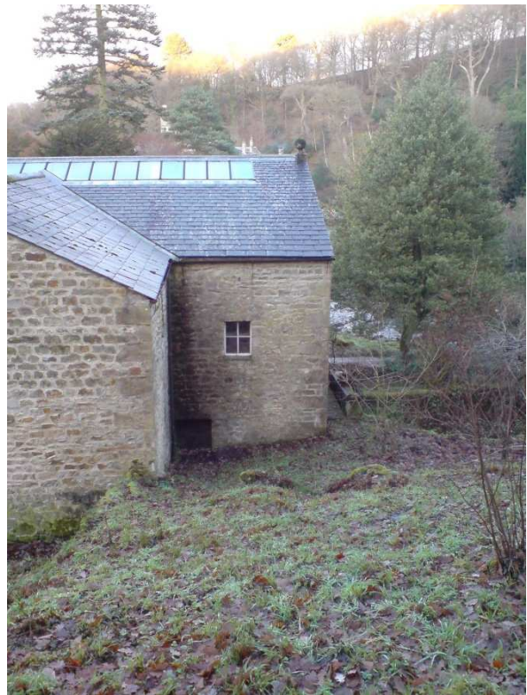
Figure 4 Gresgarth mill with the mill race running into the right hand side of the building
