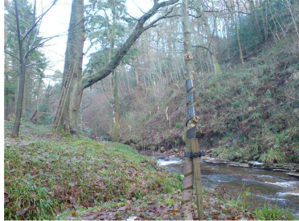
Figure 3 Location of the weir with the beginning of the leat in the foreground
