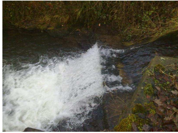
Figure 3 Top weir from above
