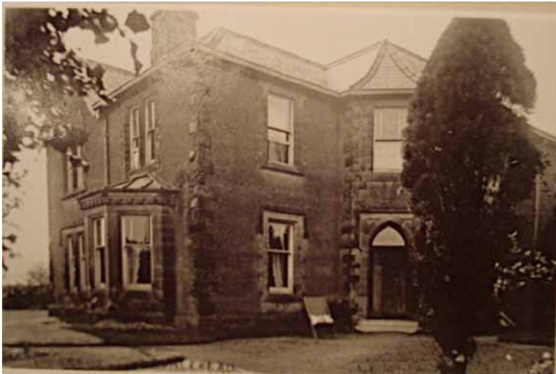
Plate 14: Vicarage, looking south
