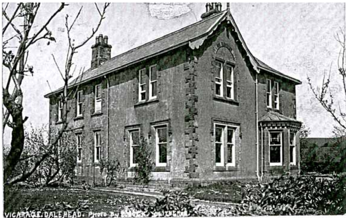
Plate 15: The vicarage, looking north
